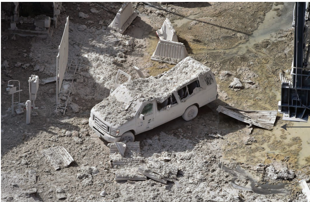
Fabric of any kind will be very little protection against the weight of debris and the sharp edge of metal sheeting.
