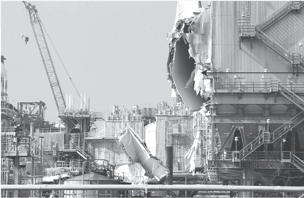
In most blast events, the heavy steel materials used onsite become projectiles and are sometimes more dangerous than the blast wave itself.
